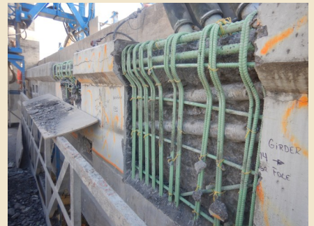
Concrete removed to expose damaged areas
