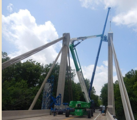
Crews reset the upper tower cap plates on the Beach Road cable-stayed bridge, June 2026.
