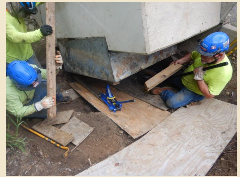
Crews inspect and reset a lower anchor cap, June 2026.
