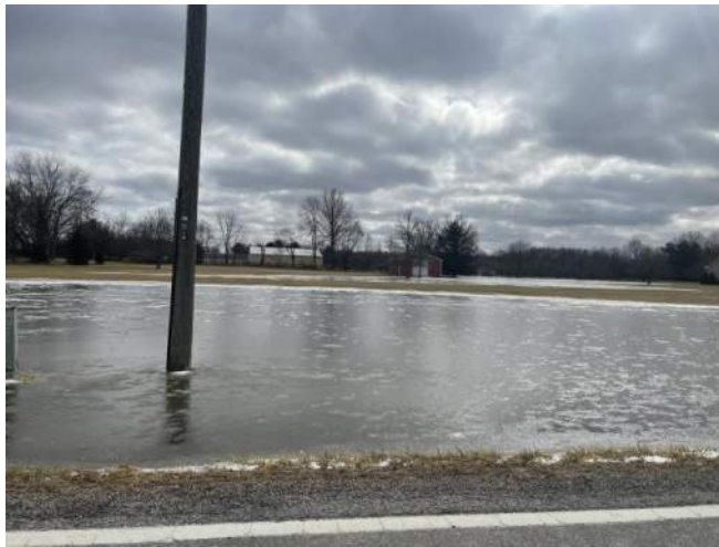
Photo 1 (8669 Patterson Rd. Frontage looking South; Area 1)
